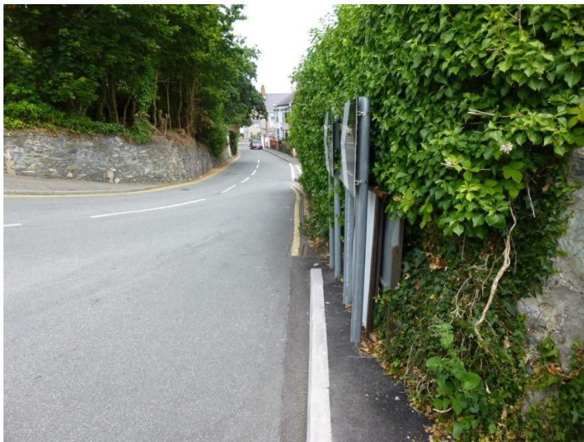
Photograph 18 – Gap in Footway Provision at Plas Road
