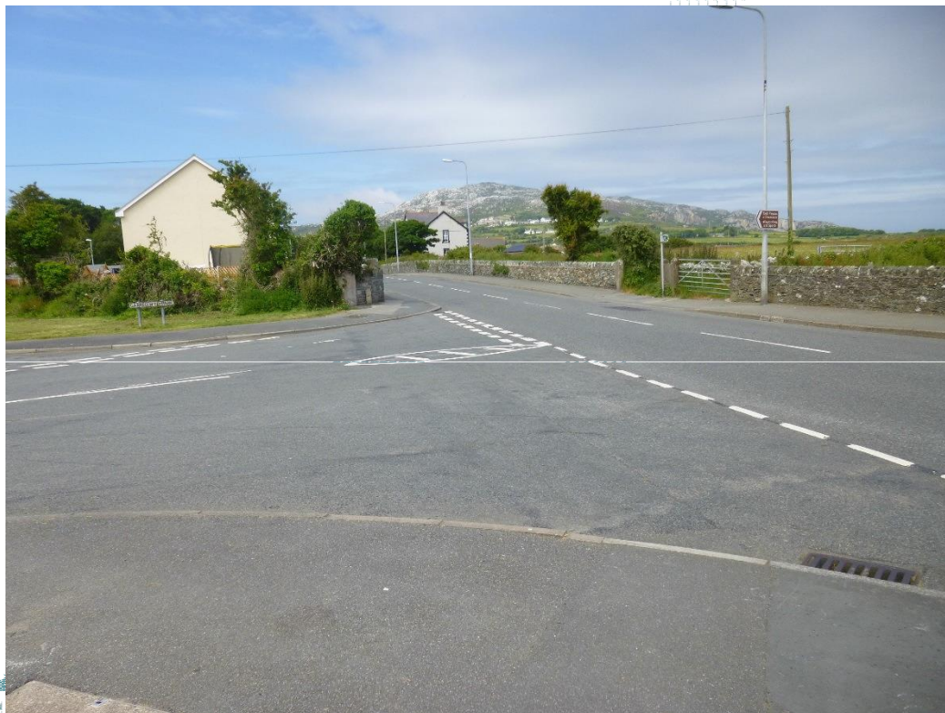
Photograph 15 - Existing Layout South Stack Road / Garreglwyd Road Junction
